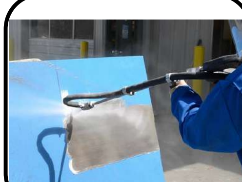
WATER SAND BLASTING
